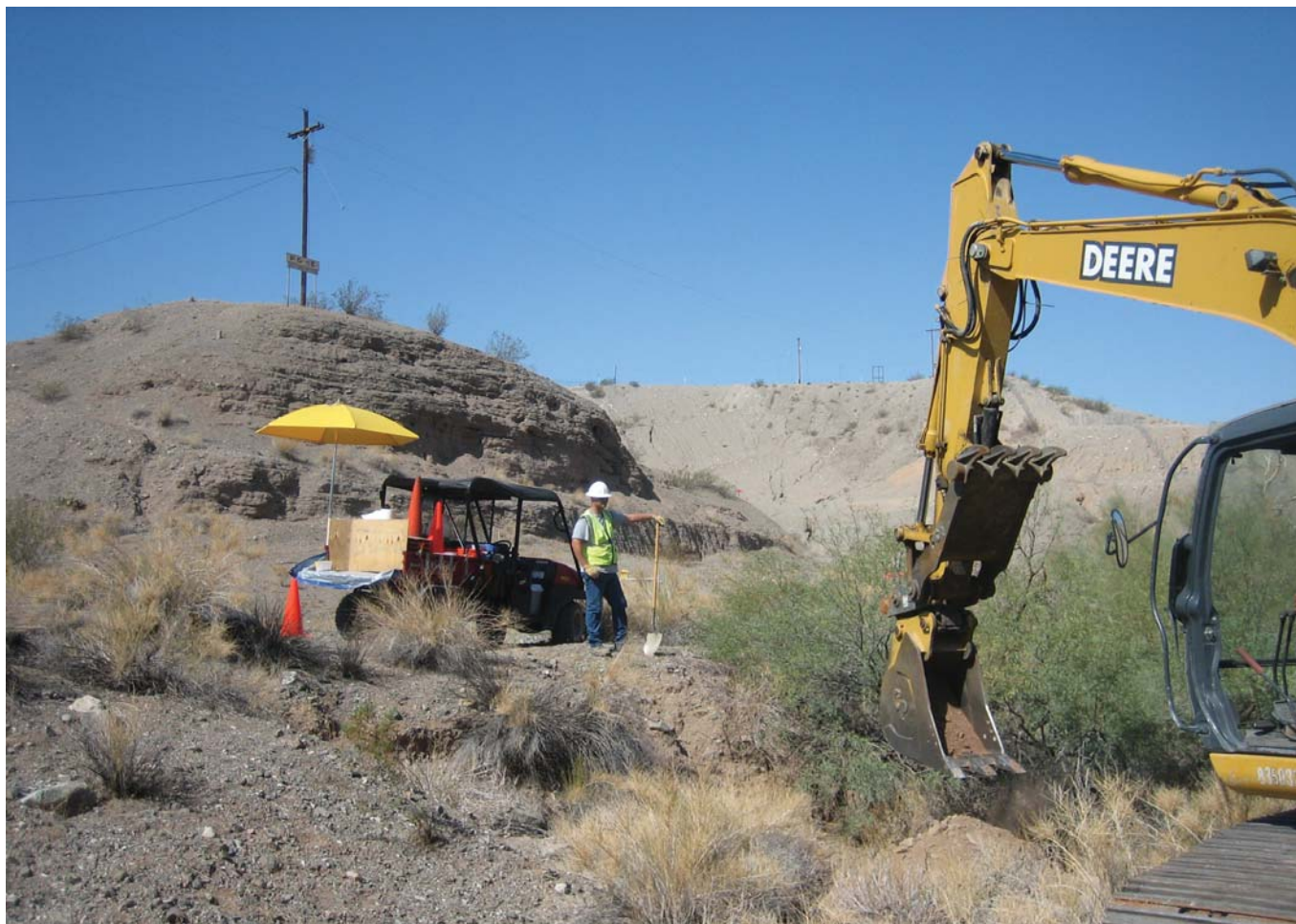
Soil sampling event at the Site in 2008 using a backhoe.
