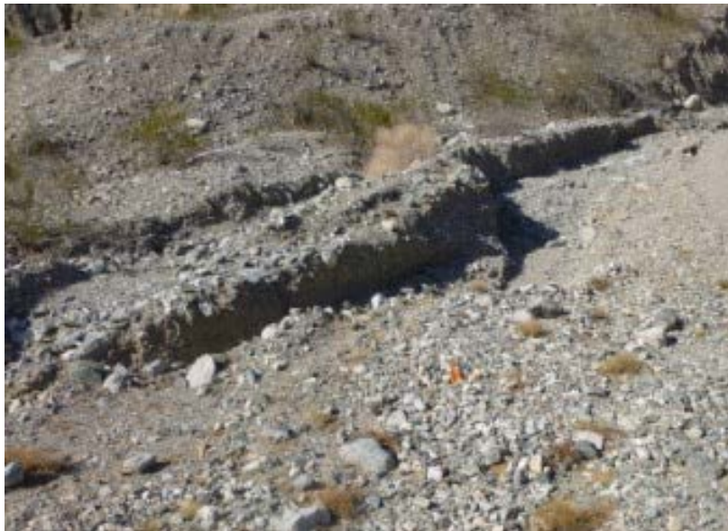
EXHIBIT 3.5-3 SEVERE EROSION OBSERVED ON ROAD, WEST OF FRESHWATER INJECTION WELL FW-2 Groundwater Remedy Basis of Design Report/Final (100%) Design PG&E Topock Compressor Station, Needles, California
