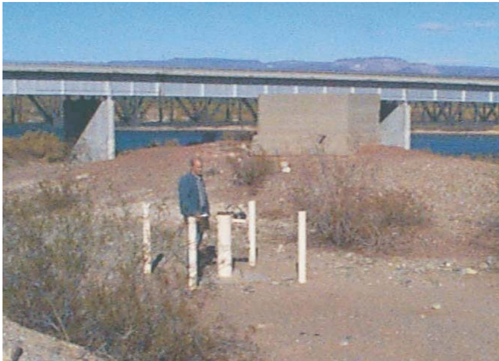
Representative above ground well completion for Floodplain site.
