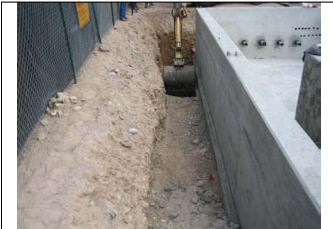
Soil removal in Valve Vault No. 1 excavation on April 28, 2005
